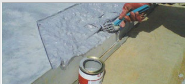
Bonding fresh concrete to existing concrete
